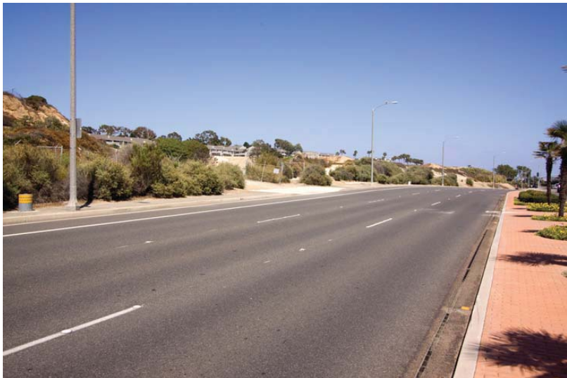
View 4 - View along West Coast Highway looking east.
